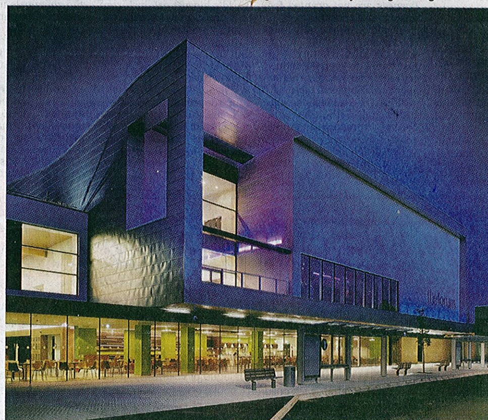
A recent electrical installation by D.E.S at the University of Hertfordshire
